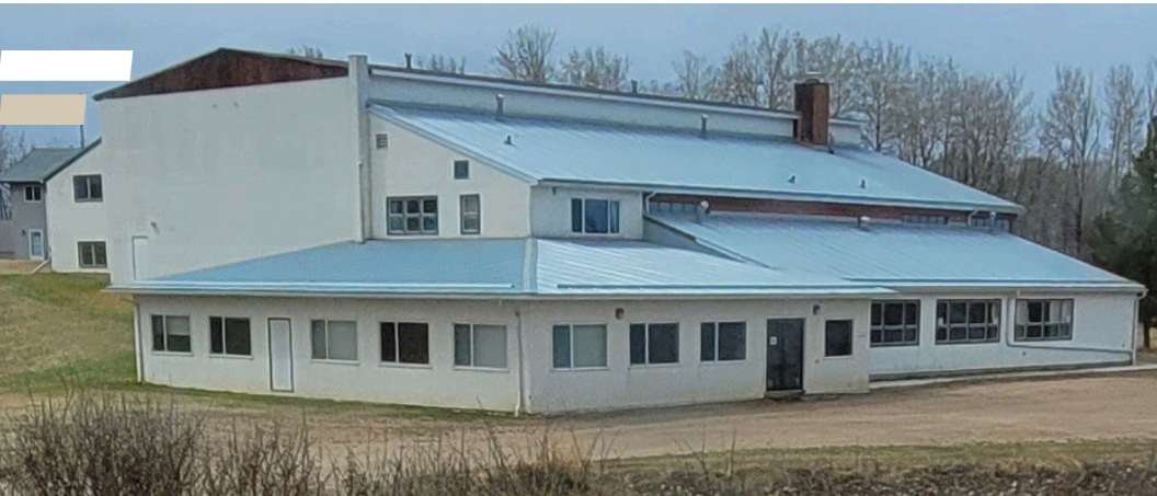
Main building of KDC
