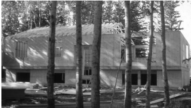
Trusses going up on house
