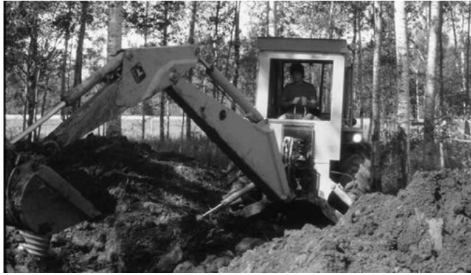
Steve did digging with the backhoe
