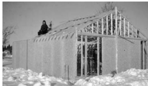
Doug building the mission hall in January
