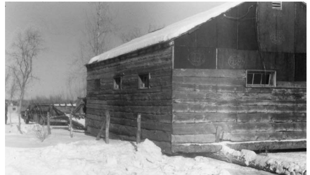
Moving the storage shed into Cumberland House
