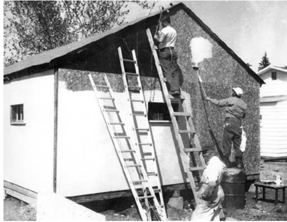
Men from Mennonite church in Rosthern do renovations
